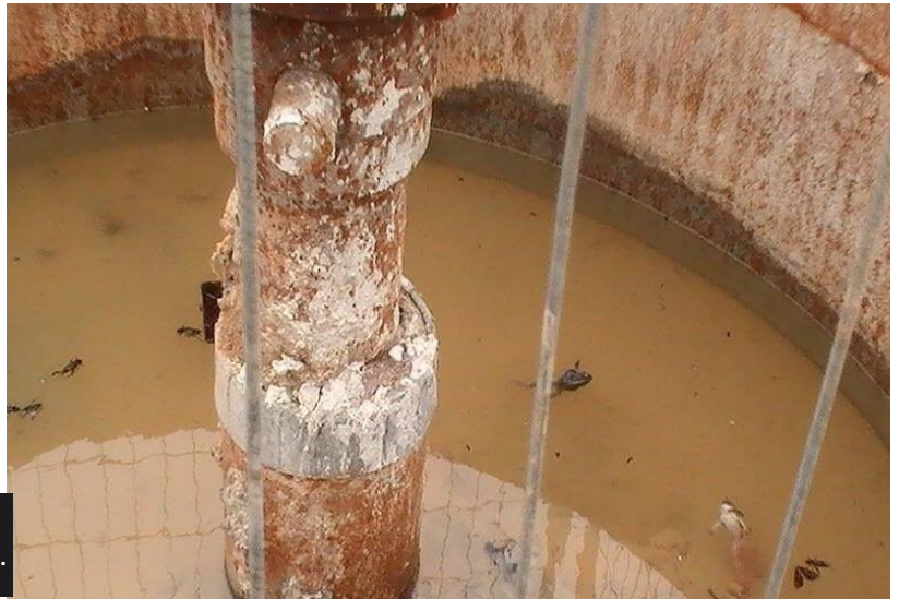
CORRODING GAS WELL in the Pilliga near Narrabri. All those dead frogs weren't too pleased with the water quality.
