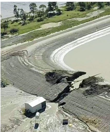
Ruptured coal seam gas holding pond in Miles QLD spews waste water onto the neighbouring farm of Joe Mills. (May 2015)
